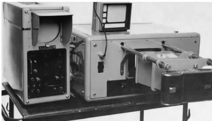
Fig. 8 Displays and camera from the bed-table scanner. Photo courtesy of the BMUS Historical Collection.
