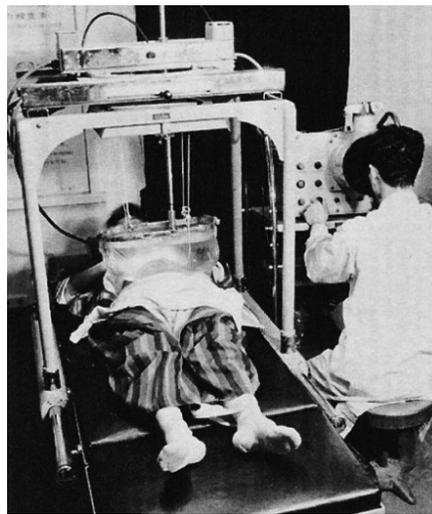
Fig. 32 The Aloka SSD-1 water-bag scanner, introduced in 1960. This was the commercial development of the system developed by the Juntendo University group (Section VIII A). Photo courtesy of the BMUS Historical Collection.
