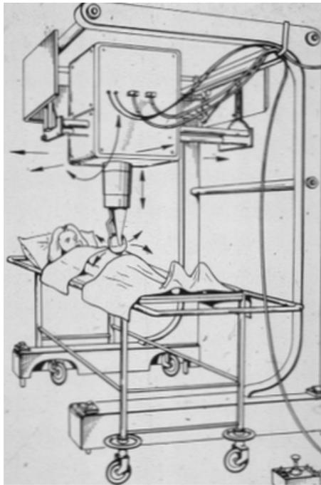
Fig. 11. Drawing of the automatic scanner from Brown [23], showing all the motorized movements. Courtesy of the BMUS Historical Collection
