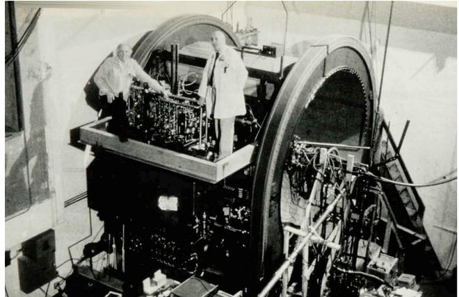
Fig. 11 Drs. Henry Blosser and William Powers on the gantry structure of the WSU/KCC FNT cyclotron during testing. (Photo courtesy of the author.)
