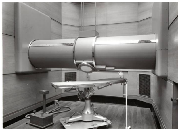
Figure 22. The 1 MV x ray tube at St. Bartholomew's Hospital immediately after installation, showing the couch and its control unit. (Barts Health NHS Trust Archives)
