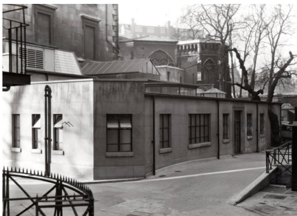
Fig 20. The north wing of the St. Bartholomew Hospital where the 1 MV “Moselle Sassoon” unit was installed. The church of St. Bartholomew the Less is visible in the background. (Barts Health NHS Trust Archives)
