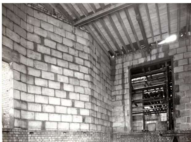
Figure 26. Photo of treatment room showing interlocking barytes bricks used for protection. (Barts Health NHS Trust Archives)
