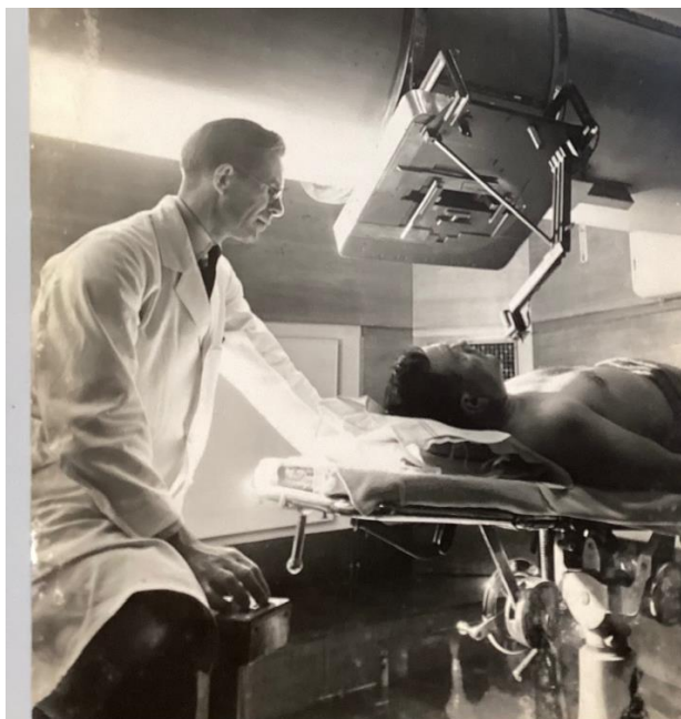
Fig 29 Dr Ralph Philips with a patient on the 1MV x-ray set. Note the mechanical front pointer to indicate the focal-skin distance. (Barts Health NHS Trust Archives)
