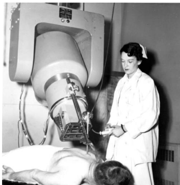
Fig 30 The Saskatoon Unit designed by Harold Johns and students, and John MacKay of Acme Machine and Electric of Saskatoon. (From University of Saskatchewan, University Archives and Special Collections)
